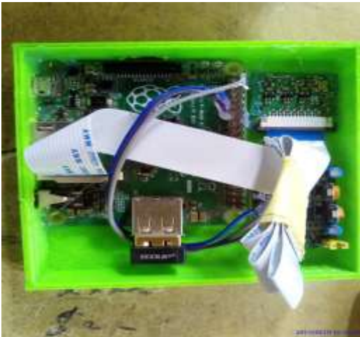
Figure 5. Smart Surveillance System Internal View
